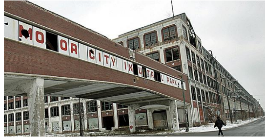
Figure 3: Packard Plant Detroit, MI
